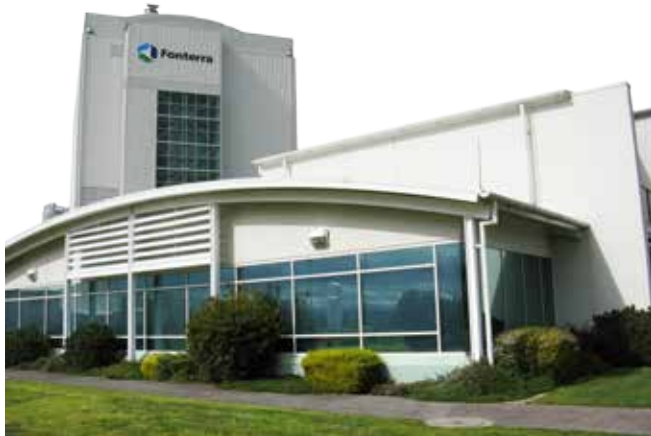
Fonterra building in Darnum, Victoria, Australia.
